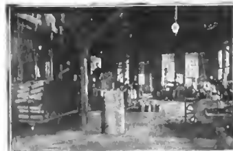
INTERIOR OF CYLINDER PLANT
